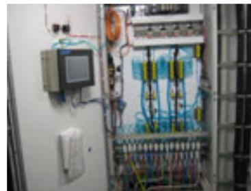
**Guard Level® Electro-pneumatic gauging for ballast, service tanks and draft point.**
